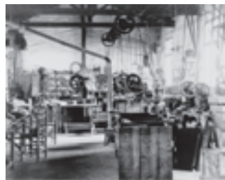
Interior of the factory on Calle Pare Roca, Olot 1925
