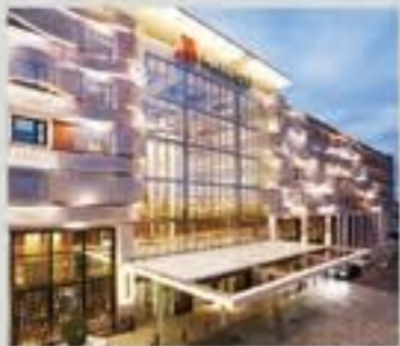
Marriott Auditorium Hotel, Madrid, Spain
