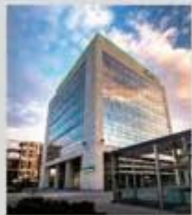
HQ Mansion of DKV, Zaragoza, Spain
