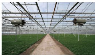
Boilers or heaters can be automatically operated during cold seasons to keep greenhouse interiors warm for stable plant growth.
