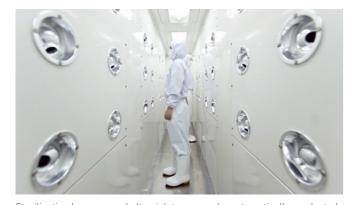
Sterilisation by ozone and ultraviolet rays can be automatically conducted several times per day.
