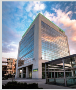
HQ Mansion of DKV, Spain
